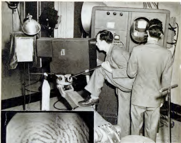
Televising a photographic enlargement of a fingerprint. Left, the print as it appeared on the screen of the receiving instrument two miles away
